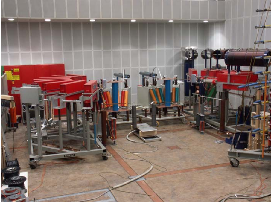
Fig. 17- Example of an impulse current generator
